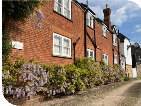
Red brick in flemish bond-
