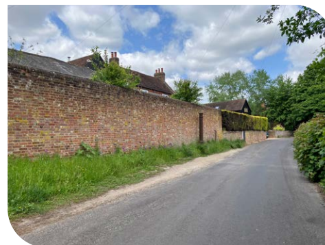
Red brick walls
