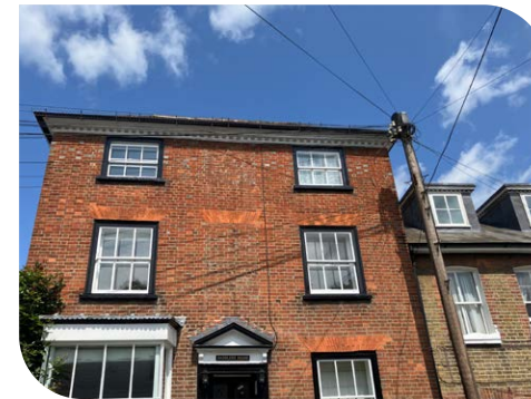
Sash windows and panelled timber door
