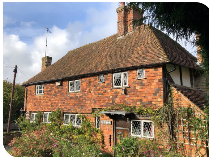
Kentish vernacular - timber framing, local red brick, tile-hanging, peg tiles on the roof and leaded casement windows
