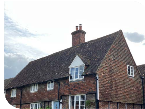
Roofs of Kent peg tiles
