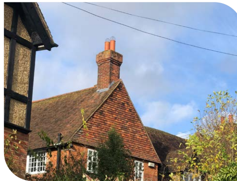
Tall brick chimneys
