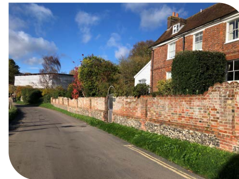
Flemish bond brickwork
