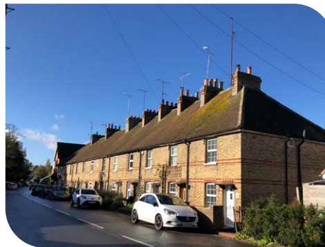
Yellow brick and clay roofs
