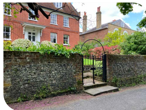
Knapped flint walls
