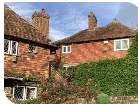
Clay tile roofs
