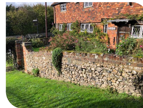
Knapped flint walls
